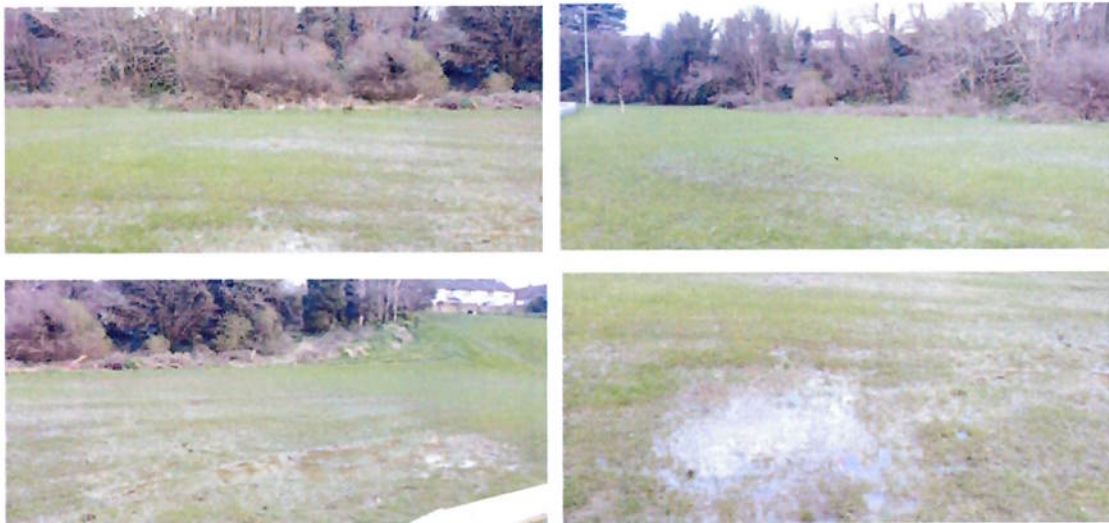
Previous construction site water-logging
